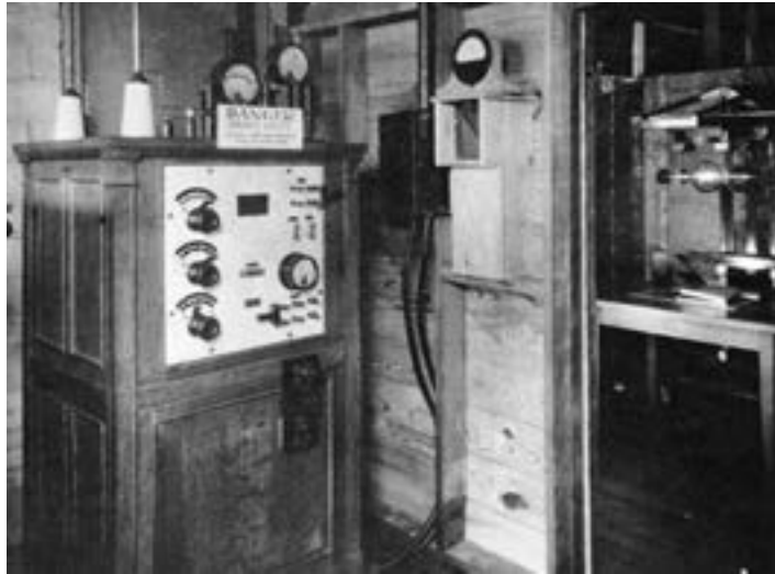
Original Materials Section - X-Ray Equipment
